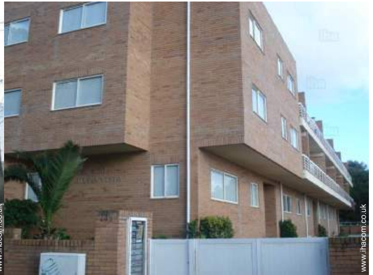
Modern block of flats
