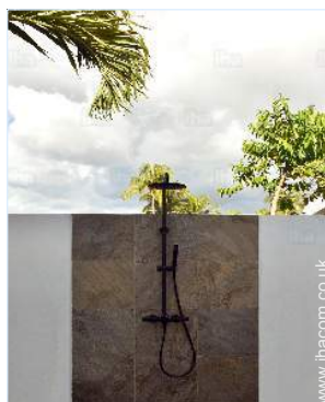
outside shower facilities
