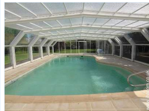
Original swimming pool
