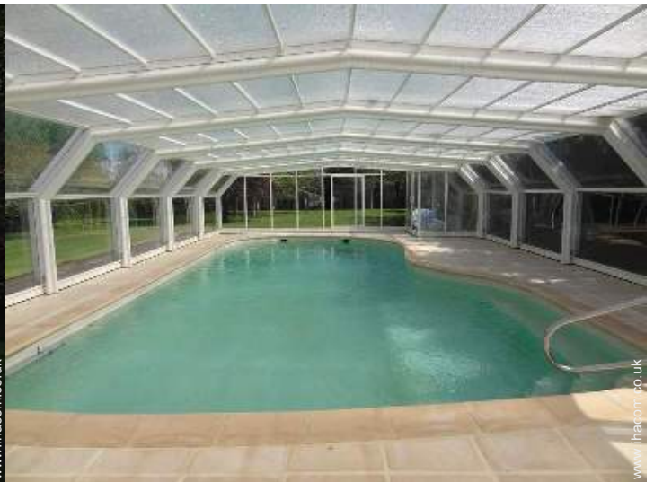
Original swimming pool
