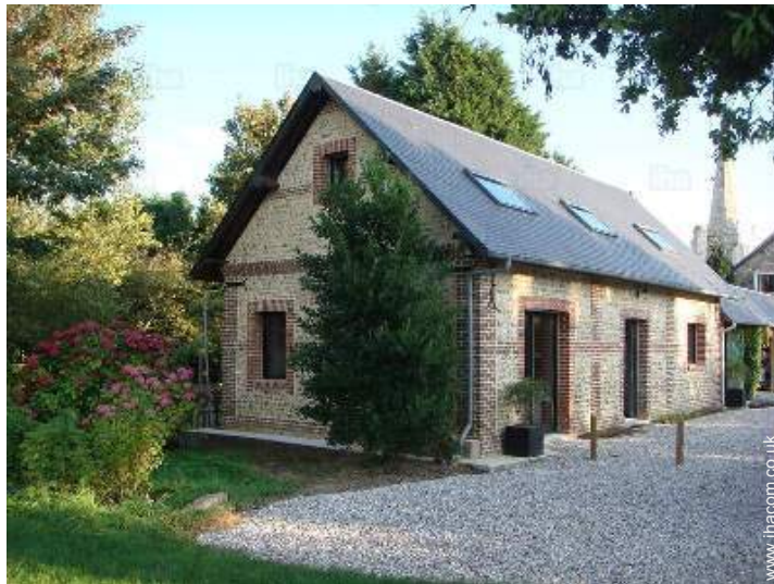
Charming Stone-Built House
