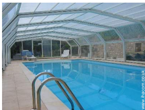
Covered swimming pool
